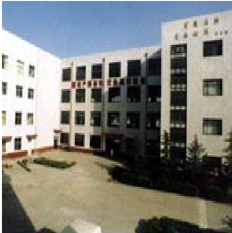
View of our factory building
